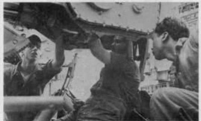
Gunner's Mate (Guns) Seaman Apprentice Scott Schepker, Gunner's Mate (Guns) Seaman Bruce Bergeron, and Gunner's Mate (Guns) Second Class Carlito Llamzon inspect the breech of one of LEAHY's 3-inch 50-caliber guns. preventive Maintenance System (PMS) is an extremely important systematic program by which ship's equipment is kept in top condition.
