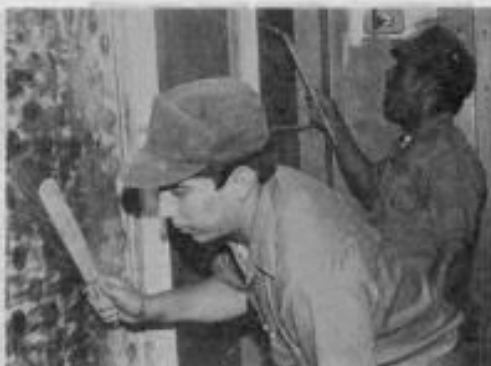
What a team! Seaman Apprentice Jimmie Jaimes sweeps down a bulkhead (Navy jargon for wall), removing dirt after chipping and grinding, while Seaman Apprentice "Tee" Manns follows right behind with a coat of primer. The final coat of paint will be applied by spraypainting.
