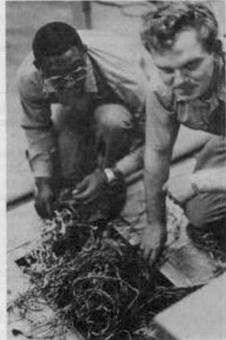
"Where do they all go?" has to be the question of Fireman Apprentice Tommy Waymyers, as the spaghetti-like maze of sound-powered phone wires are uncovered. Interior Communications Electrician Chief Kurt Djordjevic says, "I'll show you" -- and he did, checking to make sure that this vital phone circuitry was 100% complete.
