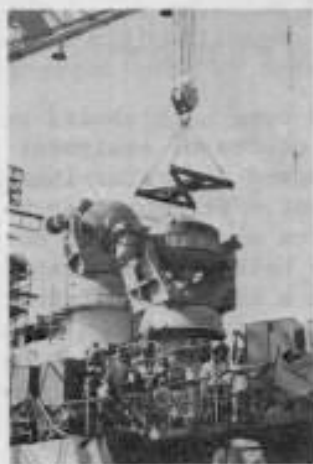
A towering pier crane eases one of LEAHY's four fire control radars onto its housing. These radars track and guide our missiles after launching to their designated targets.
