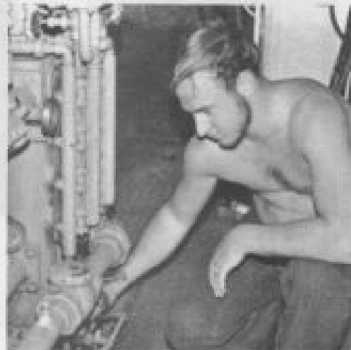
FN Taylor from Lake City, Fla. drains air lines in the fire room in order to remove moisture from the air.
