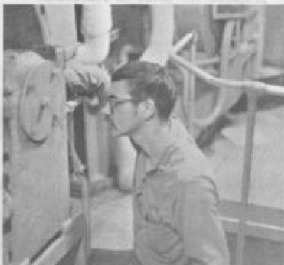
BMFN Lewis of El Paso, Texas carefully checks the electrical brushes in one of the ship's generators.
